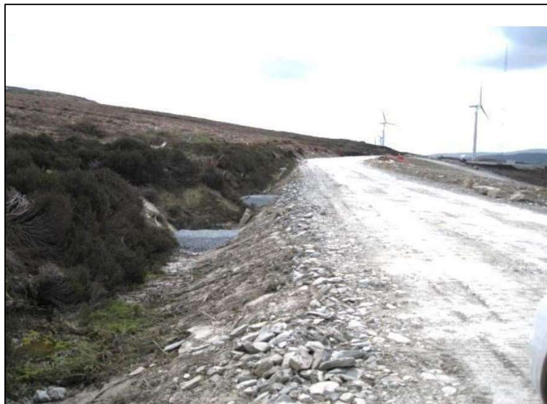
Figure 5.4 Typical example of stones used in a check dam to slow down water flow (Source: SNH, 2015) 4
