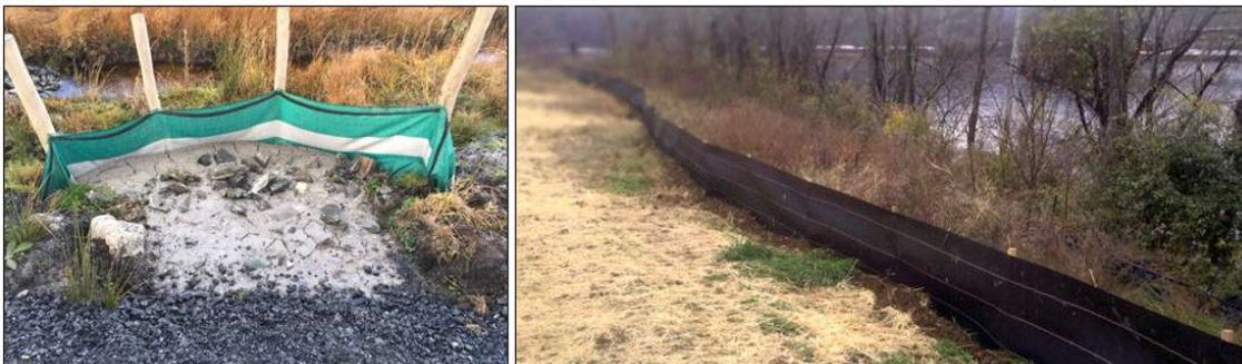
Figure 5.2 Silt fencing measures (Source: SSI Environmental (left) and Thrace Group (right))
