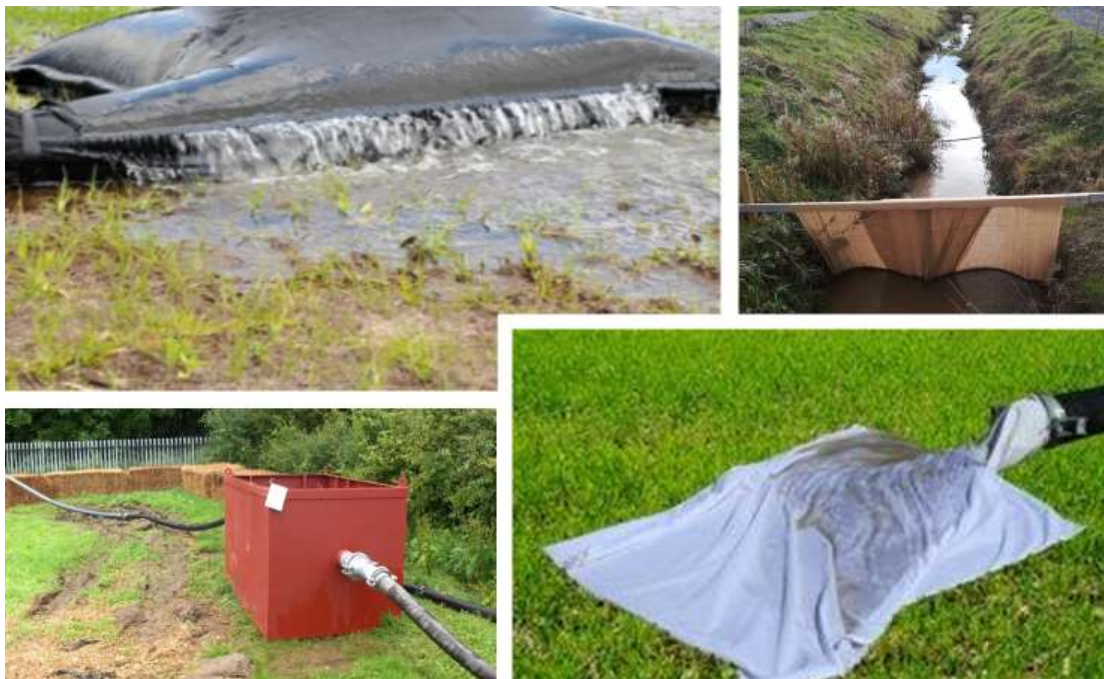
Figure 5.5 Examples of Proprietary Silt Control Measures
